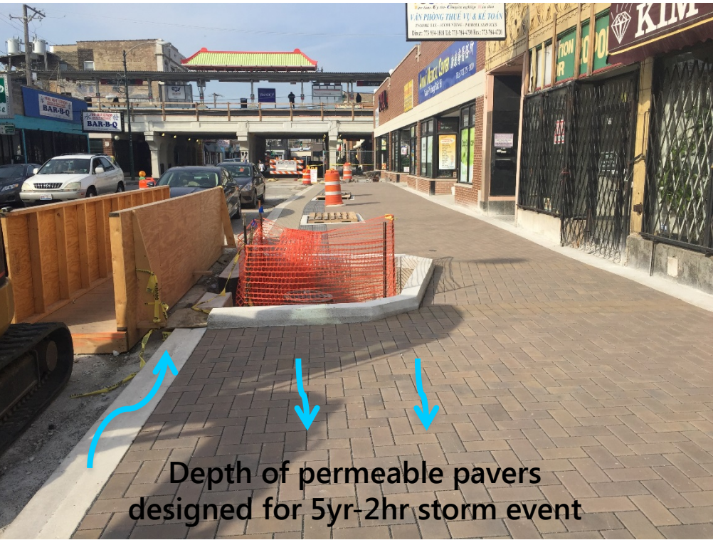
Permeable Paver Section
