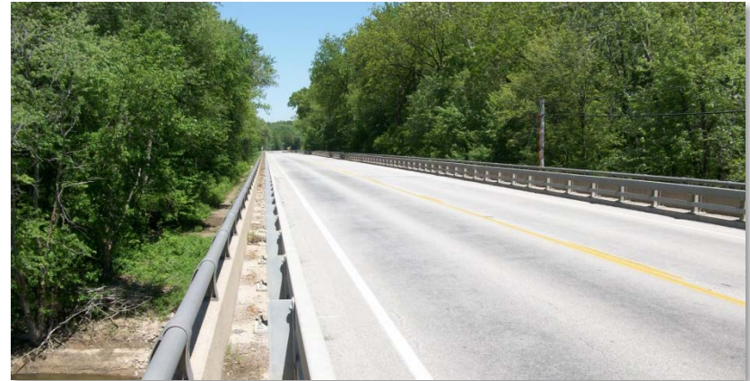
▲ EXISTING | Looking north along existing structure
