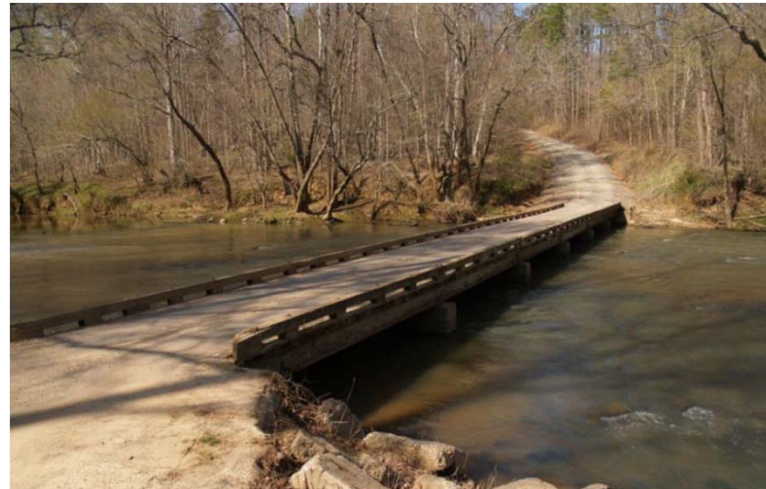
Low water bridge at Montgomery County, NC
