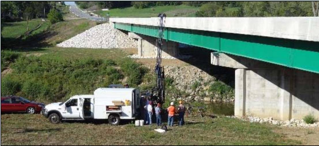
US 24 over Lamoine River, Brown County
