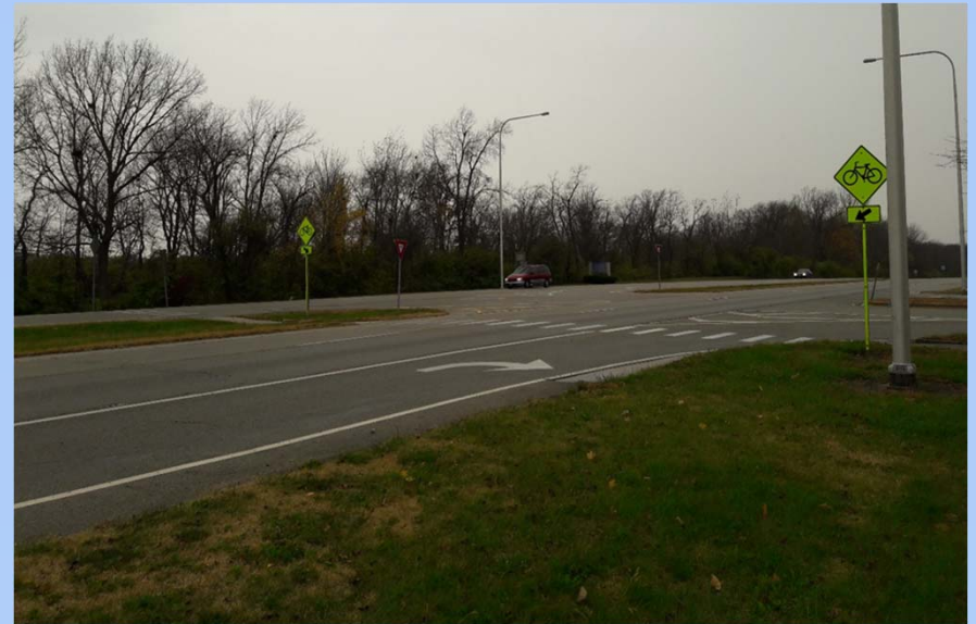
Retroreflective Signpost along IL 23, Rochester, IL.
