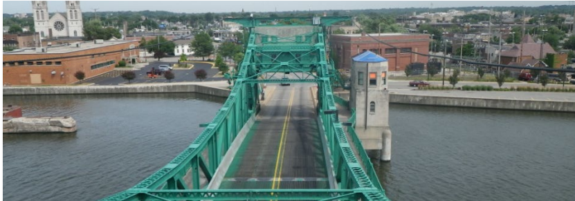
▲ Jackson Street / Bridge Street Bridge
