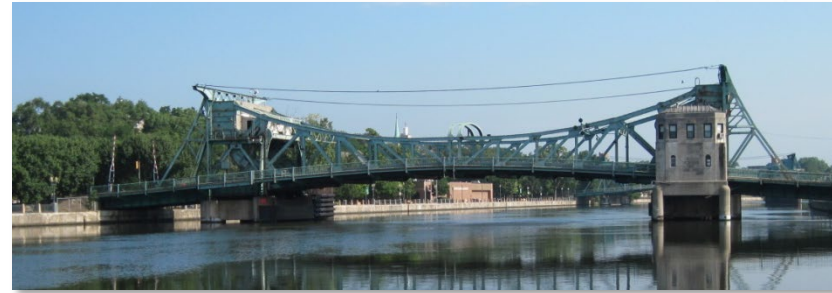
▲ Jefferson Street / US 30 Eastbound Bridge
