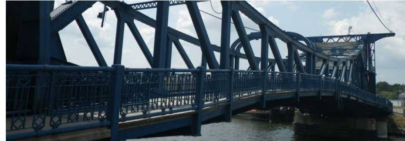
▲ McDonough Street / US 6 / US 52 Bridge
