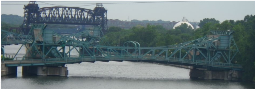
▲ Cass Street / US 30 Westbound Bridge
