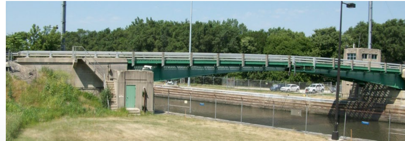
▲ Brandon Road Bridge
