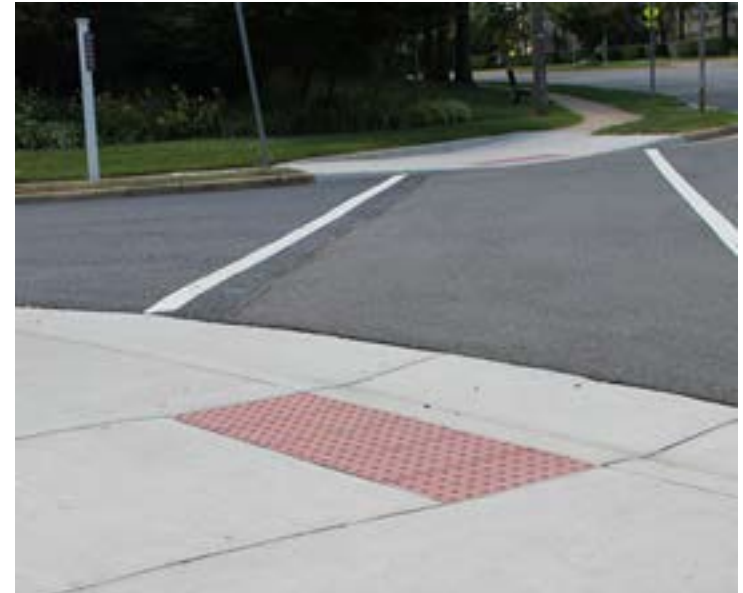
Source Accessible Curb Ramp, U.S. Access Board
