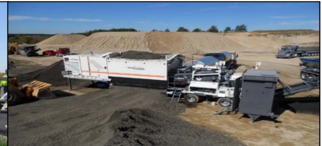
Cold Central Plant Recycle (CCPR)
