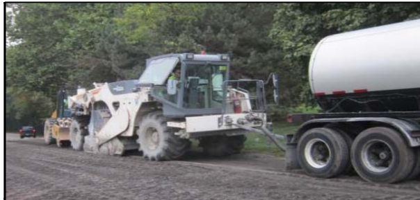
Full Depth Reclamation (FDR)
