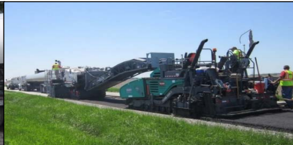
Cold In-place Recycle (CIR)
