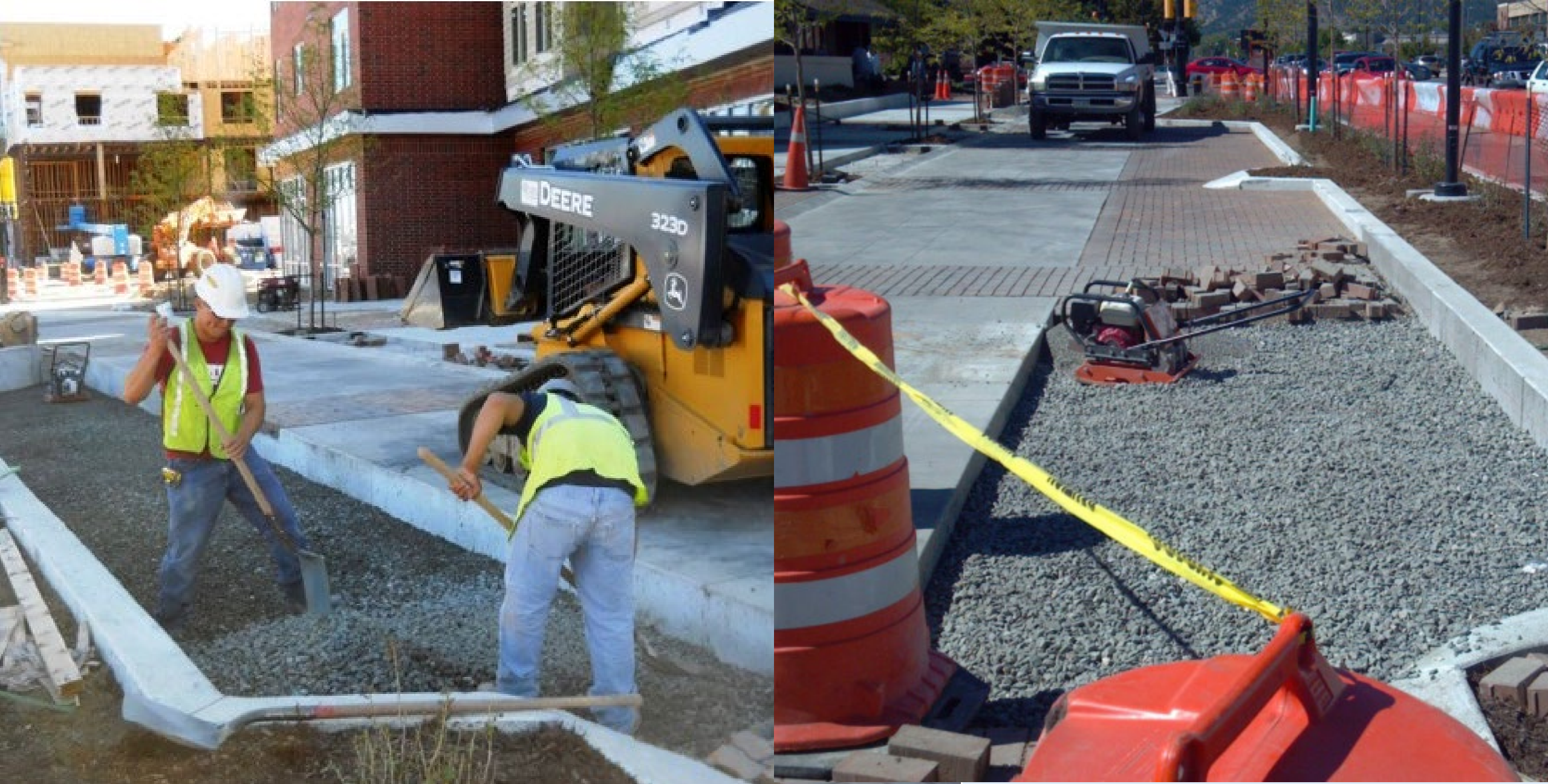
Pearl Multi-Way Boulevard: Permeable Brick Paver System
