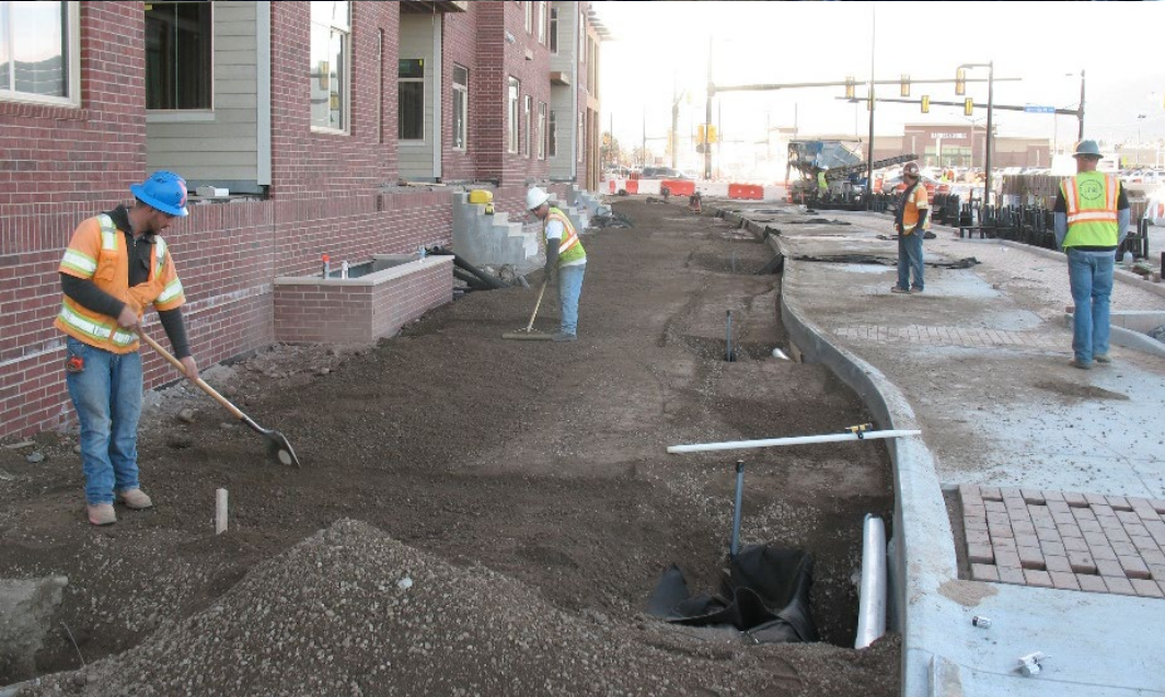
Pearl Multi-Way Boulevard: Silva Cells under Tree Strip
