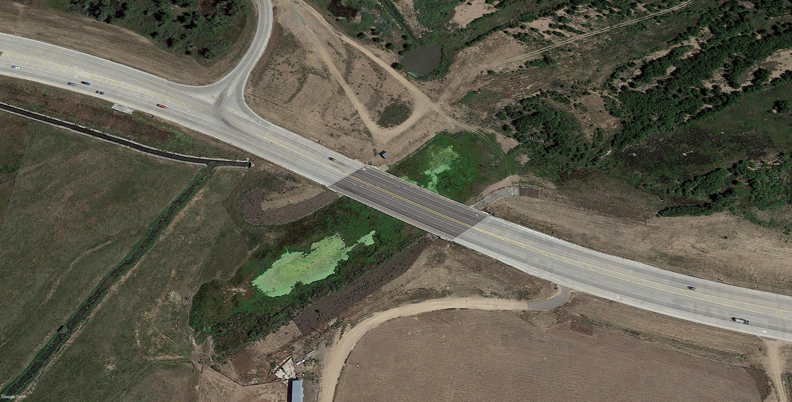
Historic 2013 Colorado Floods - US 34
