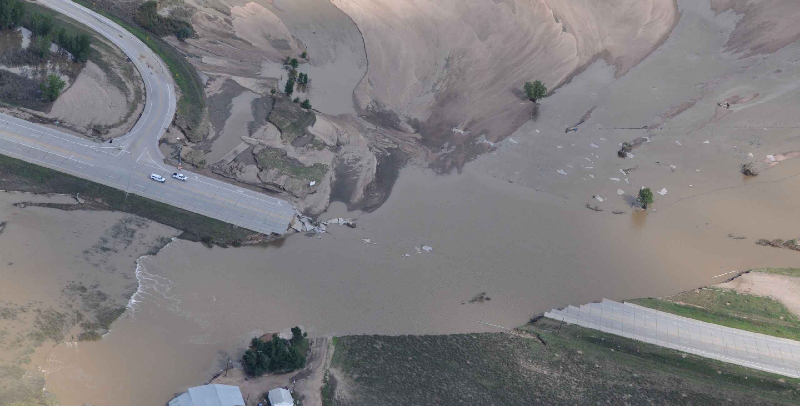
Historic 2013 Colorado Floods - US 34
