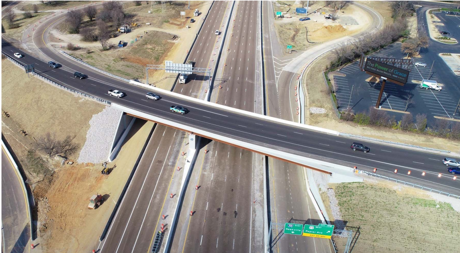
222' – 2 Span Steel Girder Bridge
