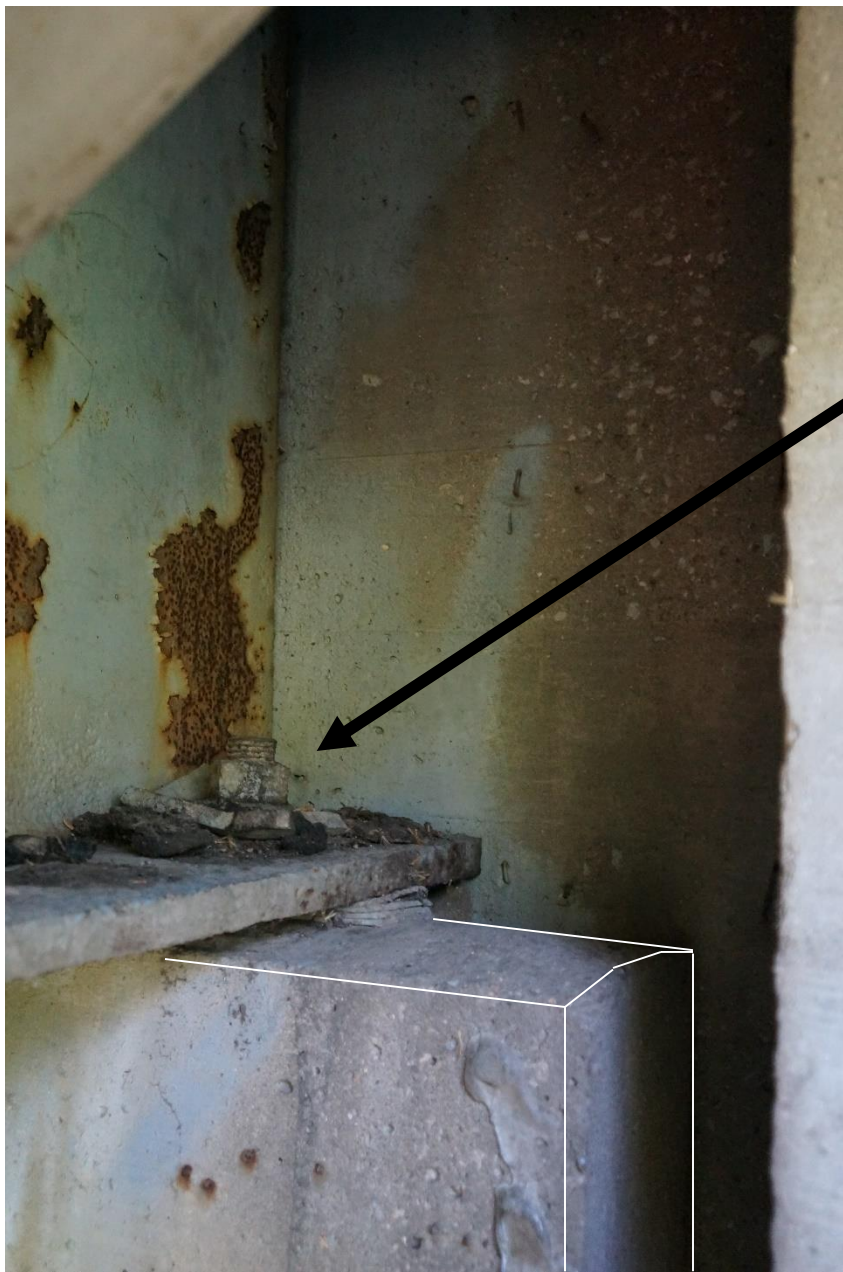
STEEL GIRDER END SUPPORTED BY CONCRETE ROCKER
