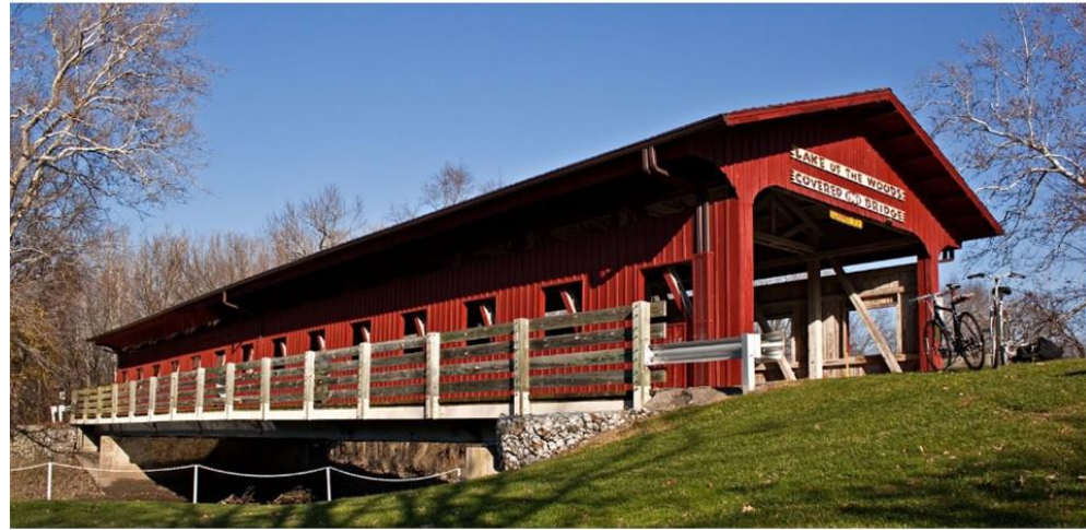
LAKE OF THE WOODS BRIDGE
