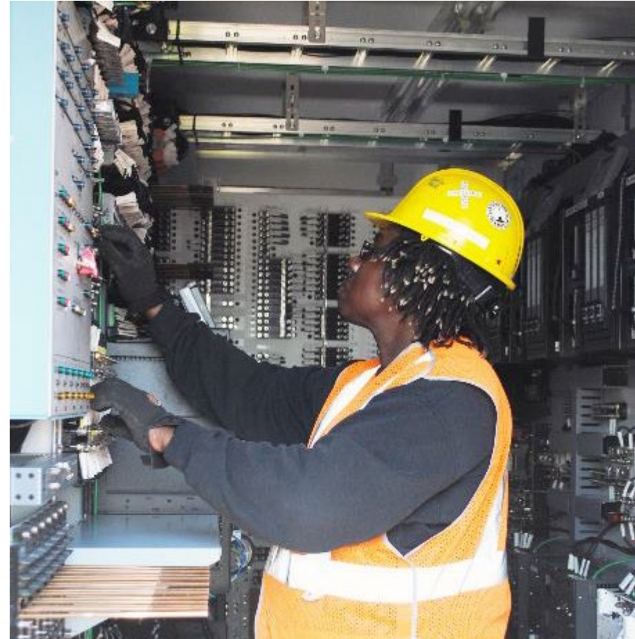
Photo taken during B1 construction
