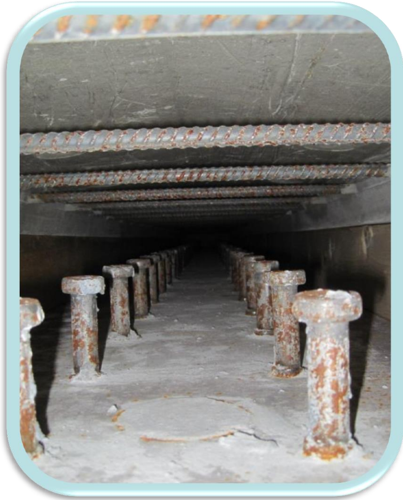
Steel Girder Connection
