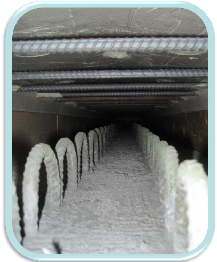
Concrete Girder Connection
