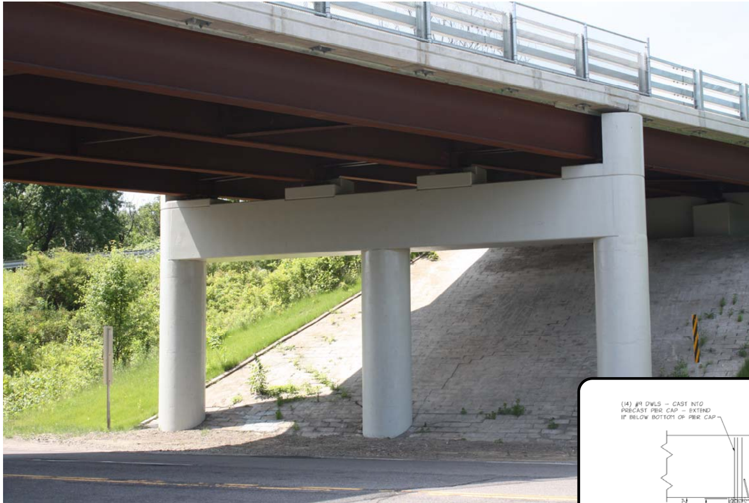
Hooper Road over Route 17C Union, New York
