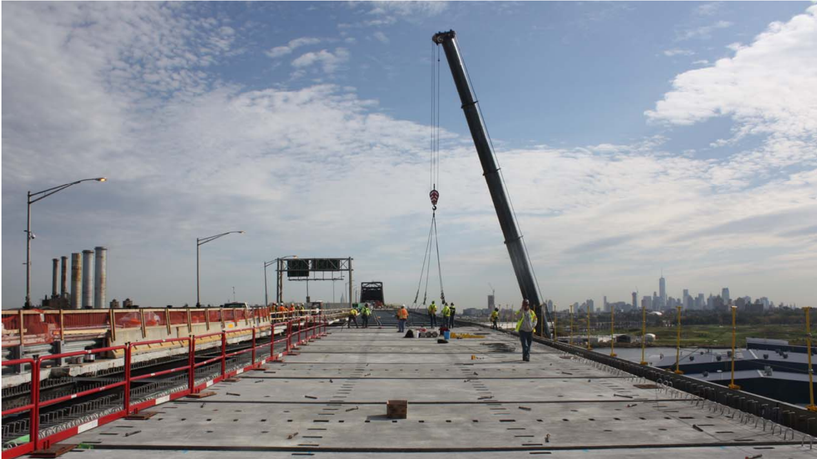
Pulaski Skyway Newark, New Jersey
