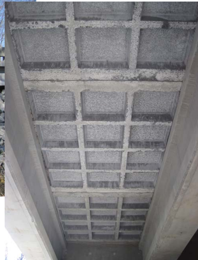
Dahlongega Road Bridge in Wapello County, Iowa
