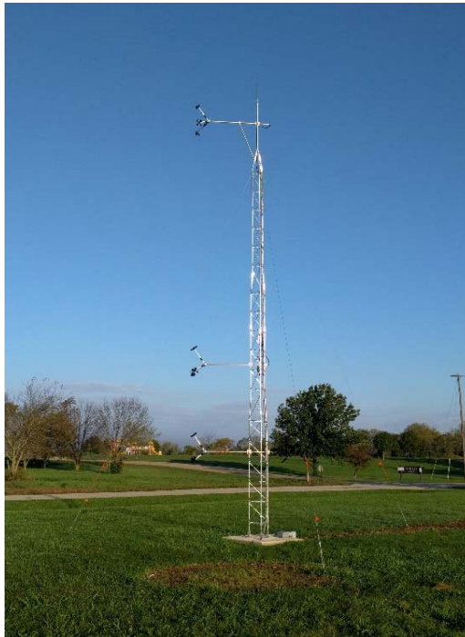
10 m Tower (Operational as of Sept. 2017)
